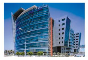
For facetted curtain walls, corner mullions are adjustable from 15° to 145° in Comar 6 and from 7.5° to 165° in Comar 6EFT. This means that roof-glazing applications, such as barrel vaults, pyramids and sloped glazing, can be achieved.
