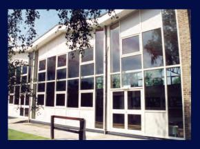
Thermally broken, Comar 2 integrates with Comar 5 to provide tilt and turn, pivot, side hung, top and bottom hung opening vents. For a full façade solution the comprehensive range of Comar 7 doors can be incorporated. Doors can be operated by overhead, concealed closers incorporating an anti-finger trap for protection. If automatic doors are required, Comar's unique door beams offer aesthetically pleasing finished applications.
