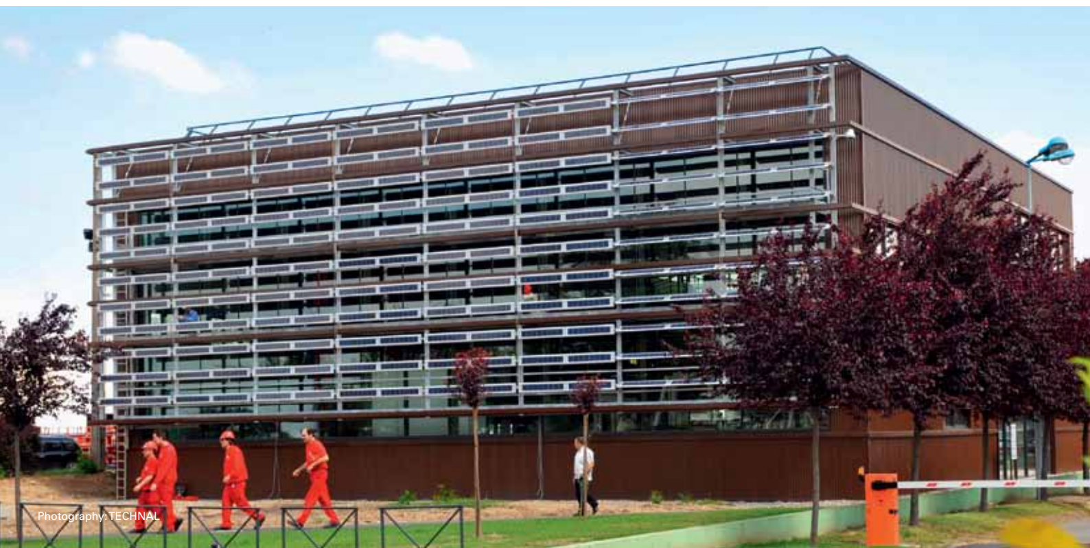
Attached to a self-supporting structure independent of the facade
